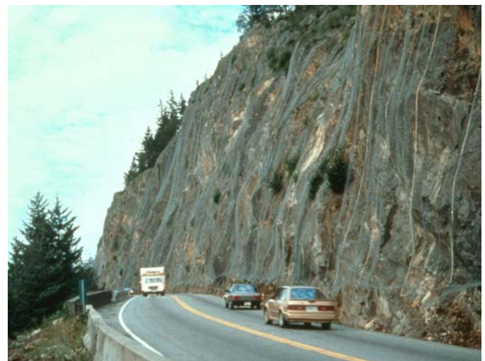
Example of Rockfall protection netting
