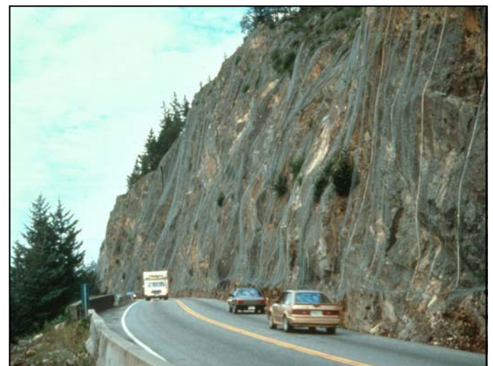
Example of Rockfall protection netting
