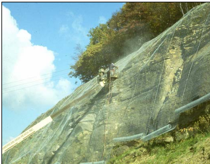
Example of Rockfall protection netting
